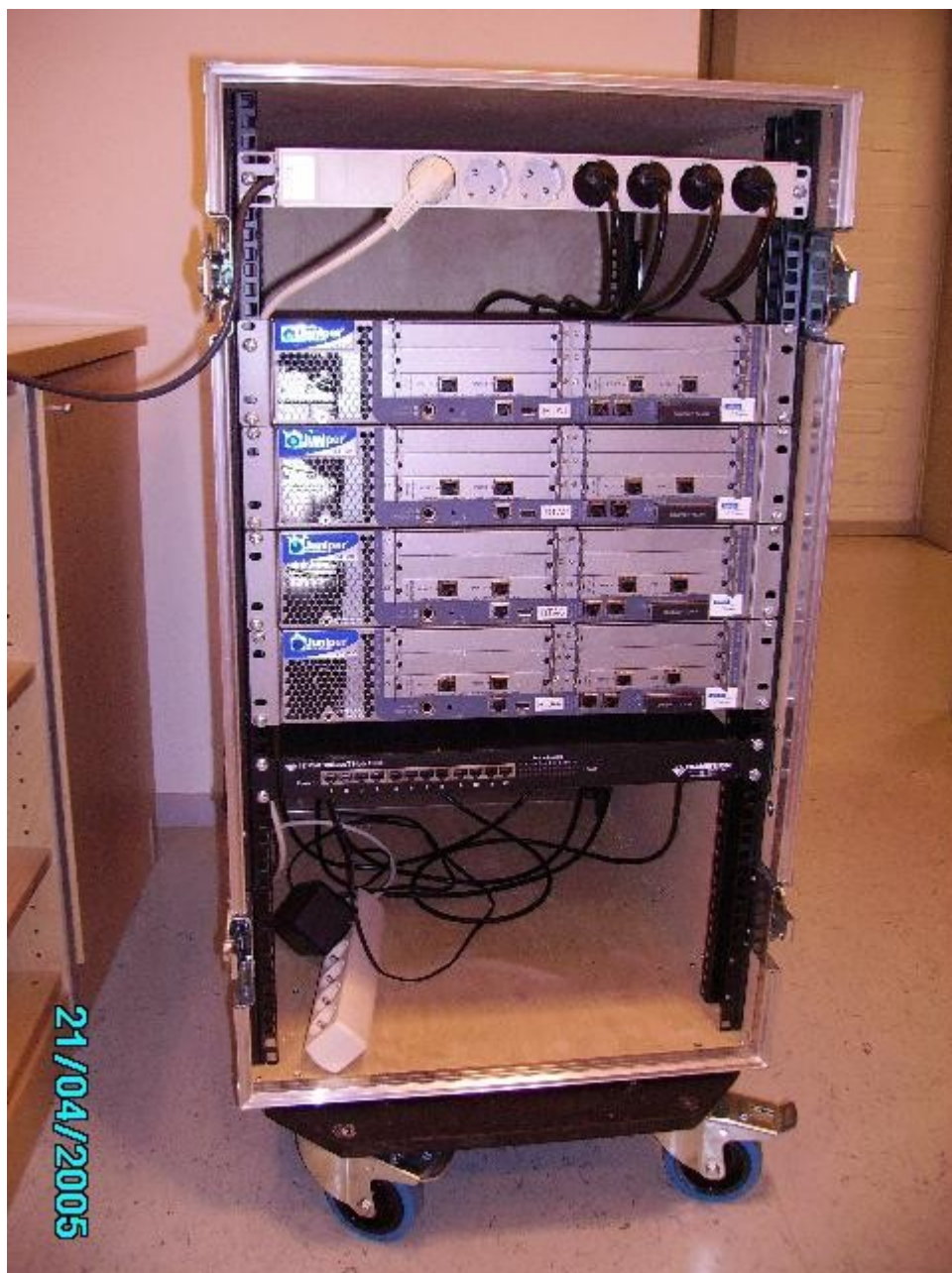
Figure 1: Mobile rack with four Juniper routers, one power panel and a hub.
