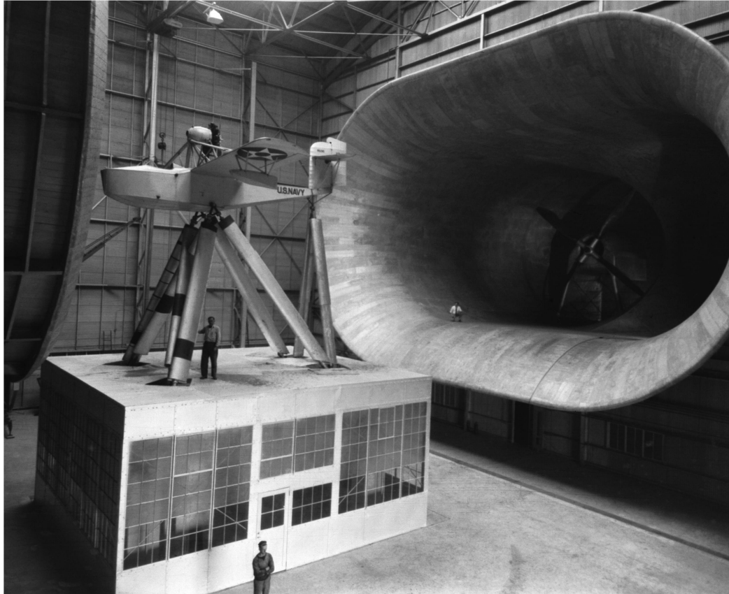
Figure 12.1: Langley full scale wind tunnel 1931: Entrance and exit cones with people showing the dimensions.
